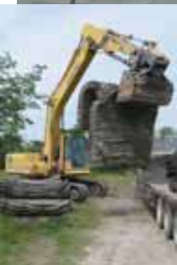
Blast mats, made from recycled tires, are now being draped over the clay dikes to stop erosion. They are transported to their dikes by - truck, backhoe, and barge.
